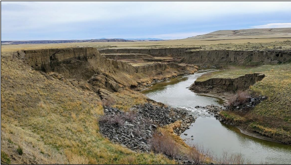
Photo 3-2. View downstream of lowermost sill at RM 3.15; note mass failure on left bank and erosion on right.
