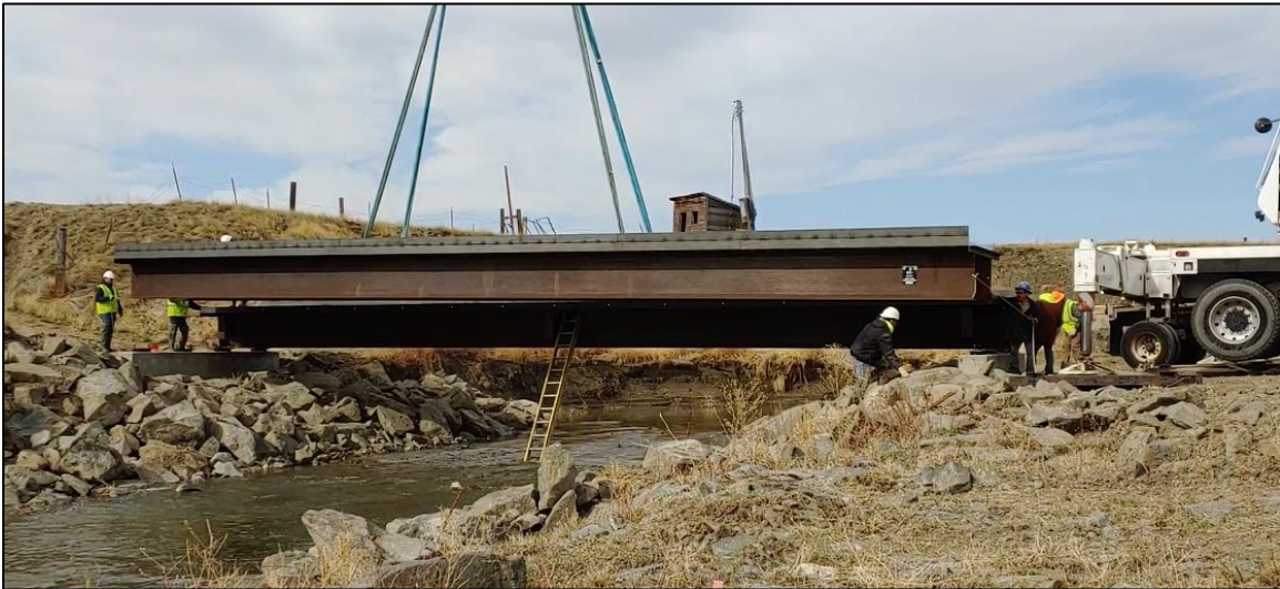
Photo 4-5. View upstream of the bridge placement following culvert removal.
