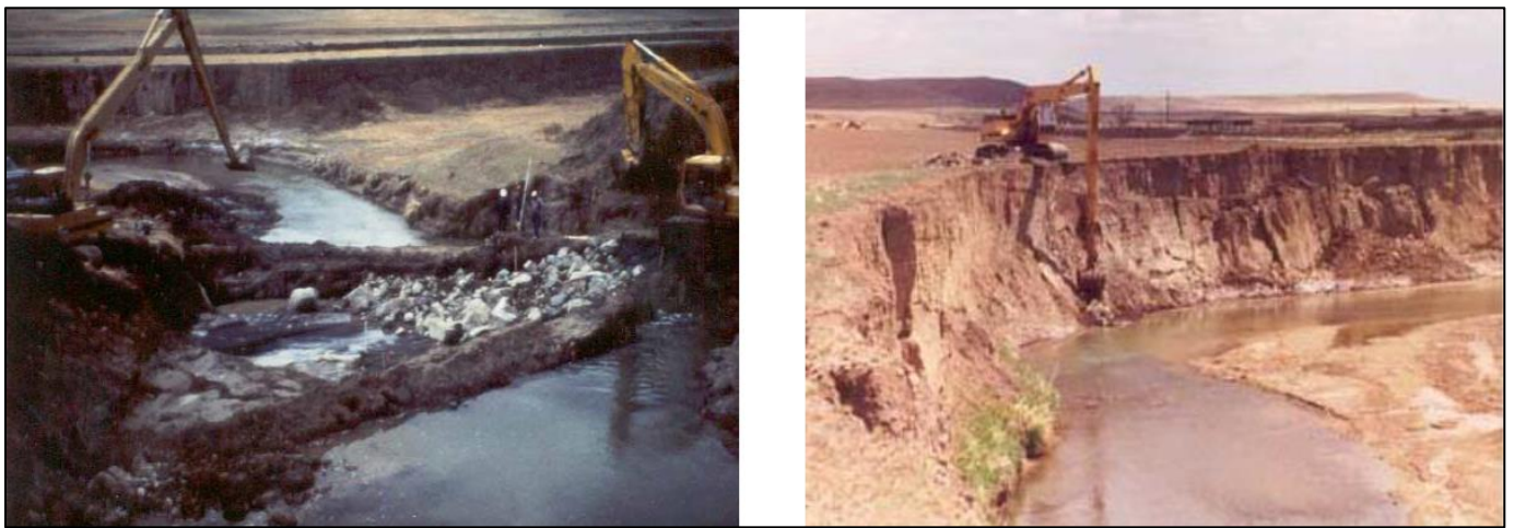
Photo 3-1. Demonstration project including rock drops (left) and barbs (right) constructed on Muddy Creek in the early 1990s.
