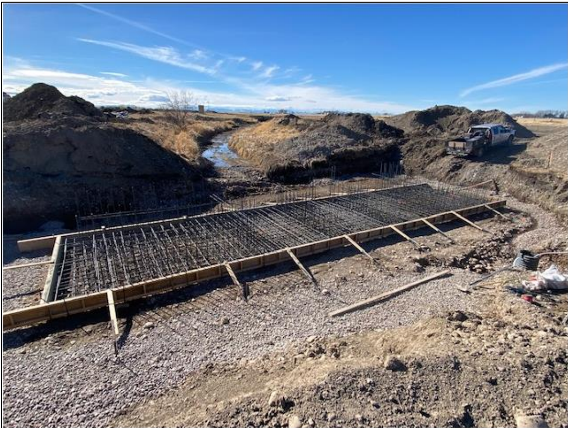
Photo 4-3. Foundation slab construction at Spring Coulee Headworks on March 22, 2022 (E. Juel).
