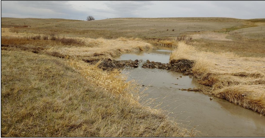
Photo 4-6. View upstream of 2022 project work on Spring Coulee showing rock drop designed to stabilize grade, increase diversity, and improve floodplain access.
