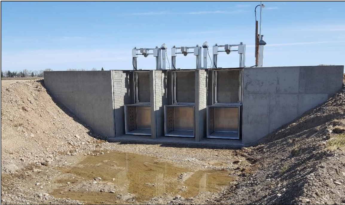
Photo 4-1. New smart headgate at head of GM-100 at J-Wasteway outlet, Spring 2020 (E. Juel).
