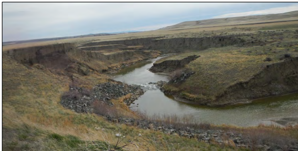
Photo 1, April 29, 2021. View downstream showing Muddy Creek drop structure within incised channel.
