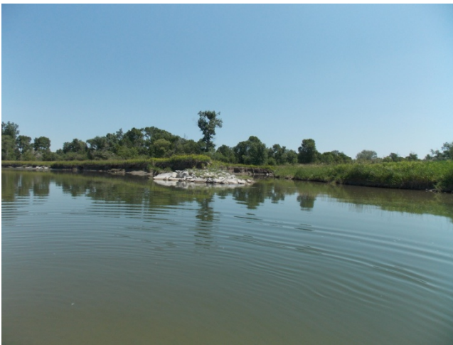
Point #1: Looking downstream at the hard point that separates the Sun River mainstem (left) from the side channel (right). Rock was placed to create this hard point over 10 years ago. It was repaired in late 2013.
