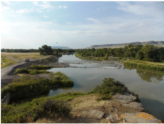
Site photos of the Rocky Reef Diversion taken during the summer of 2013. The diversion backwater creates a wide cross-sectional area and low velocities. A large amount of gravel and silt have deposited upstream from the diversion.
