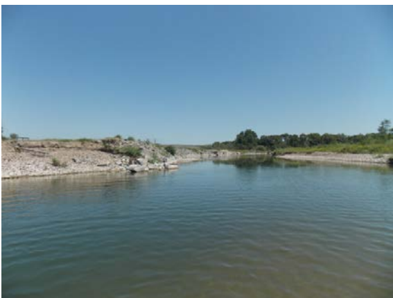
The upper end of Site SR-15. The river has eroded over 50 feet behind the jetty. Most of the erosion occurred during the 2011 flood.
