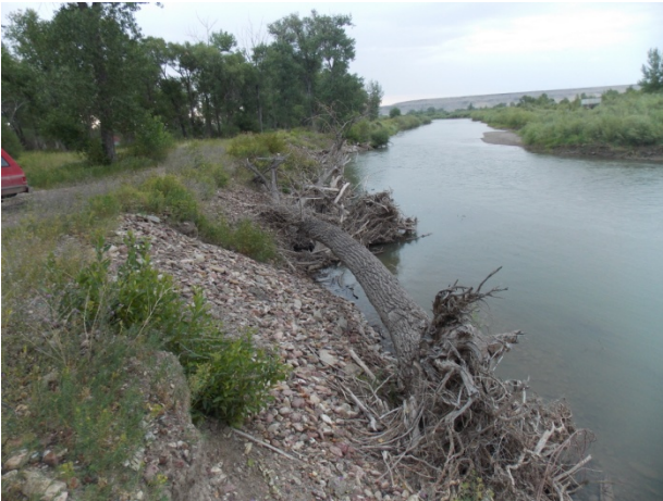
Site SR-38: Cobbles dumped over the bank serving as bank stabilization.
