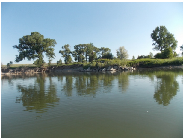
Large rock jetty that has created an upstream eddy. The eddy is eroding the bank on the upstream side of the jetty.
