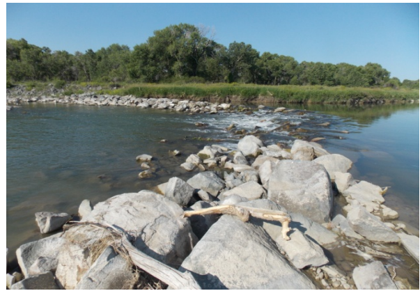
Site photos of the Rocky Reef Diversion taken during the summer of 2013. The diversion backwater creates a wide cross-sectional area and low velocities. A large amount of gravel and silt have deposited upstream from the diversion.
